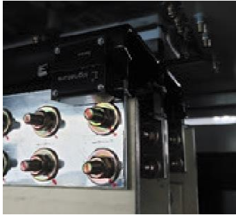
LS Cable & System Donghai Plant Busduct
